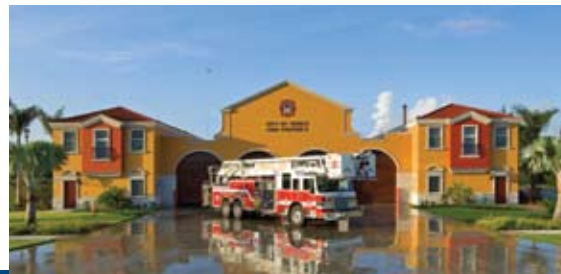
City of Venice Fire Station 3 N. Venice, Florida
